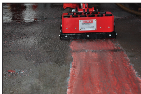
REMOVAL OF ANTI SKID COATINGS
