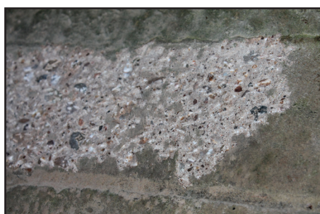
ROUGHENING CONCRETE
