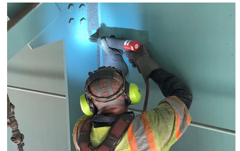
CORROSION REMOVAL
