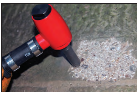
REDUCING LEVELS ON CONCRETE
