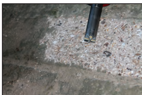
ROUGHENING CONCRETE
