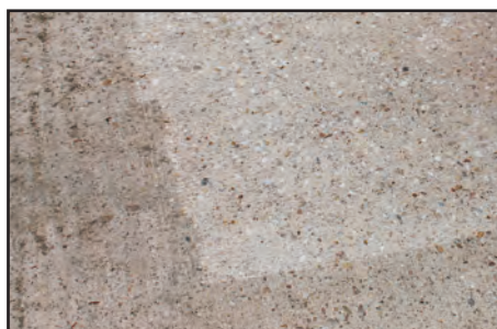
ROUGHENING CONCRETE
