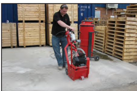
REDUCING LEVELS ON CONCRETE
